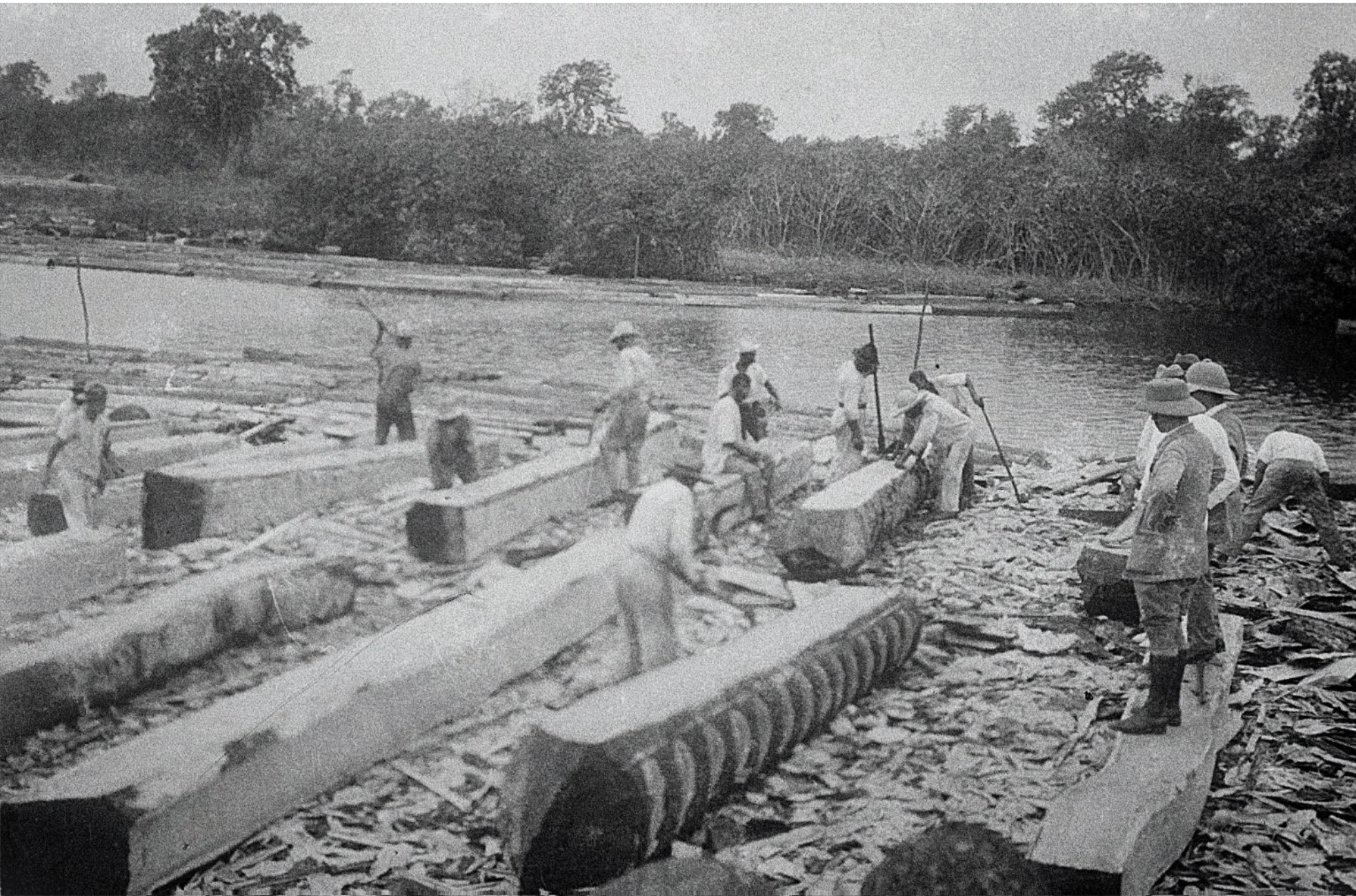
Squaring logs. Belize Estate & Produce Co. barquedier, Belize. (NSS)
